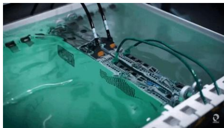
Fig. 8. Hardware submerged in dielectric fluid: LIC in practice.
